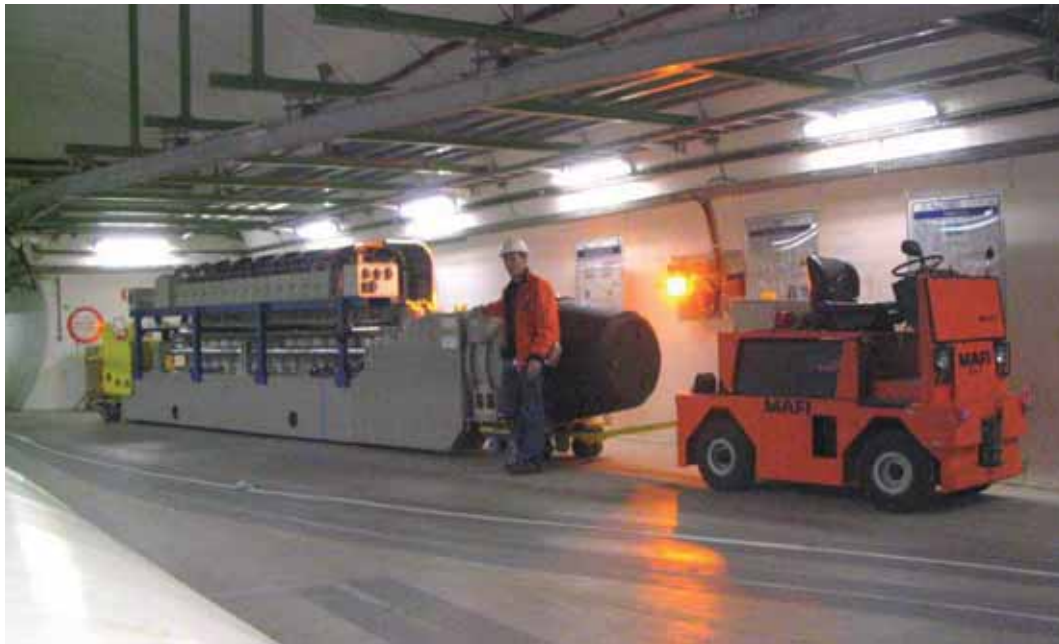
Fig. 5.1.2.1: Example of transport convoy during DFB installation at LHC.
