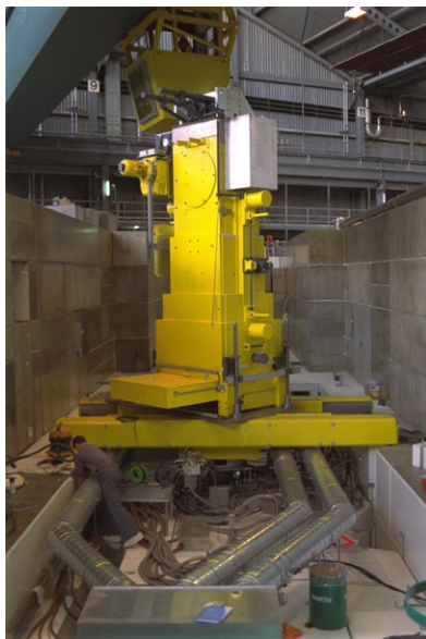
Figure 9.34: Exchange flask target E on the bridge.
