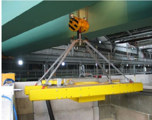
Figure 9.36: Bridge lifted by the 60 t crane.
