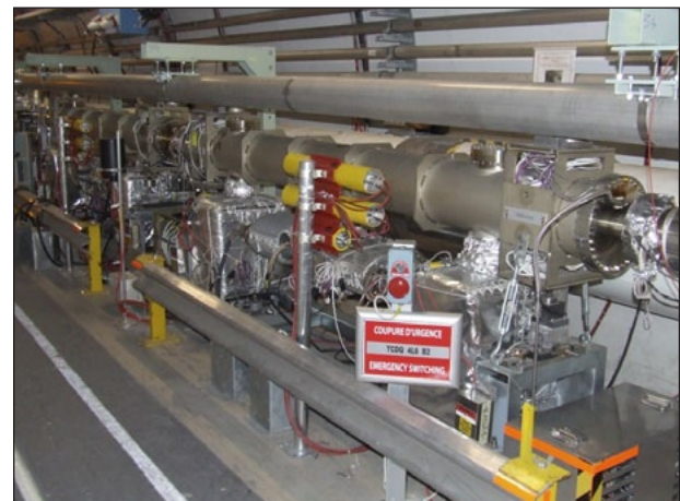
Figure 1: A view of the TCDQ assembly in the LHC tunnel (by courtesy of CERN)
