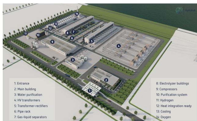
Figure 31: Visualization of a 1 GW green-hydrogen plant, based on an advanced design by (ISPT, 2022).
